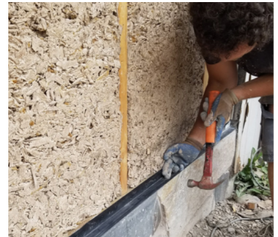
Close up of insulation made of wood chips mixed with straw and hemp fiber.
