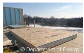
TBS continuous insulation assembly with external wall sheathing.
