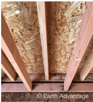
Utilizing advanced framing techniques with staggered studs.
