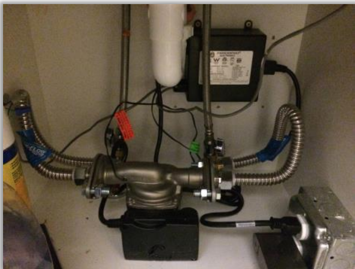
Controls a single (X1) load or pump model TLC-X1-115
