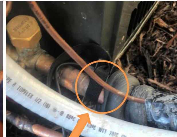
Temperature Sensors Used Instead
